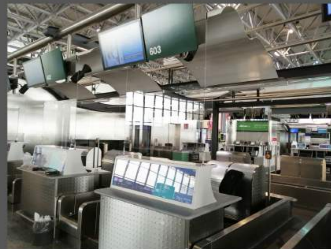
Installation of two 93x80 cm methacrylate panels.
