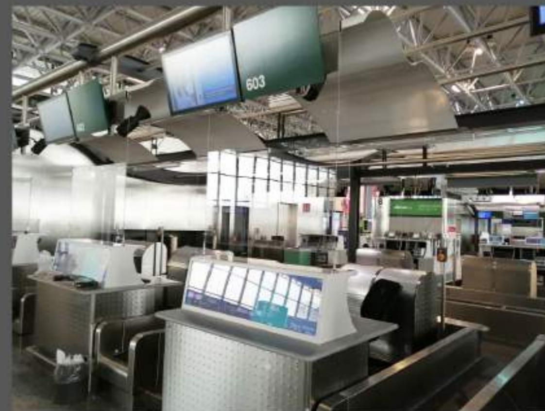
Installation of two 93x80 cm methacrylate panels.
